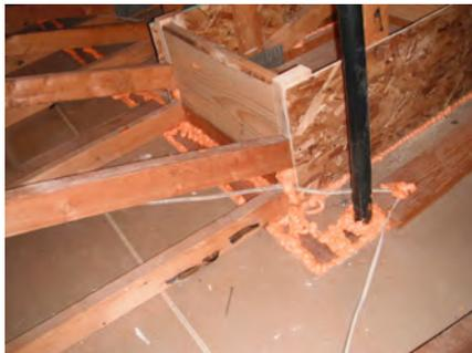
Air-sealing and insulation dam at attic hatch
