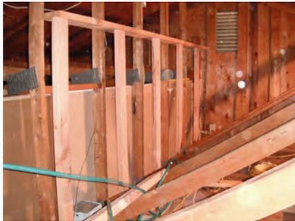
Increasing the knee wall to 8" thick and extending the height by 2' to dense pack with cellulose, then add an air-barrier over the knee wall. (the height is so the loose fill cellulose installed on the vaulted ceiling does not taper off)
