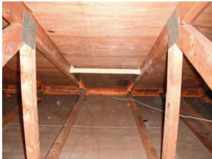
Installed air-baffle at eve vent and air-sealing
