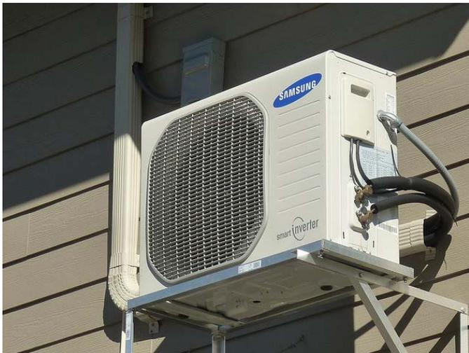
The outdoor unit of a mini-split heat pump can be mounted to the wall (above) or placed on the ground. (Source: *Gary Cziko*)
