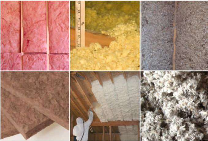
Clockwise from top left: fiberglass (batt), fiberglass (blown-in), cellulose (dense-fill), cellulose (loose-fill), foam (blown-in), rockwool
